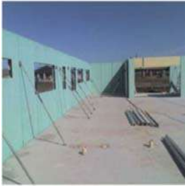
Fig. 8 Diagonal bracing Fig. 9 Corner connection
